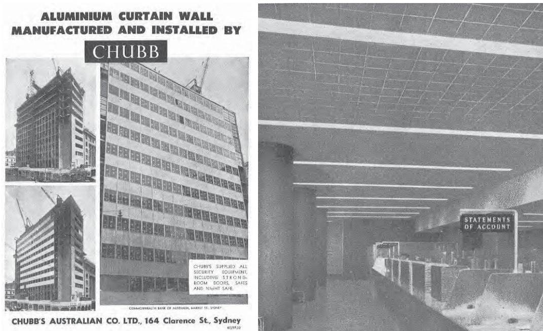
Figure 32 Chubb Australia's curtain wall system installed on the Market Street facade of the Commonwealth Bank Building (left) and Wunderlich Ltd's suspended acoustic ceiling system installed above one of the banking chambers inside the building (right). Source: Building, Lighting & Engineering , November 24 1956, pp.52 and 59.
