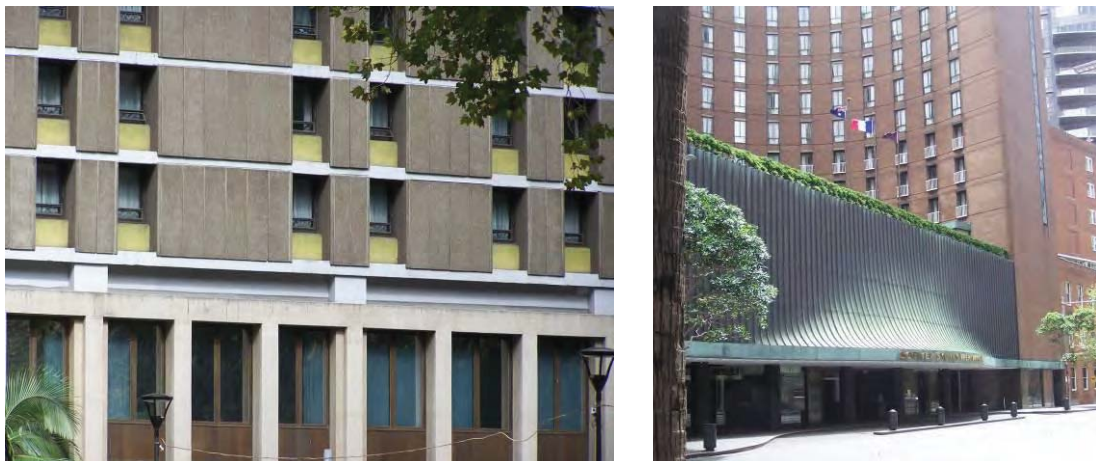
Figure 71 The rational precast concrete facade detailing of Menzies' Hotel (left) contrasts with the dramatic sweep of the light court and canopy of the Wentworth Hotel (right). Source: Roy Lumby.
