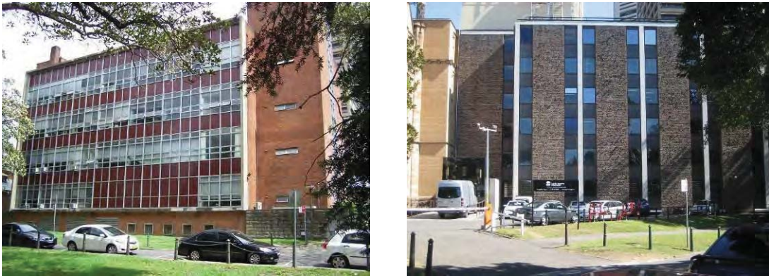
Figure 41 The Supreme Court Hospital Road Court Complex (left) and Registrar General's Department's Records Wing (right). Source: Roy Lumby (Law courts); TKDA (Registrar General's Department).
