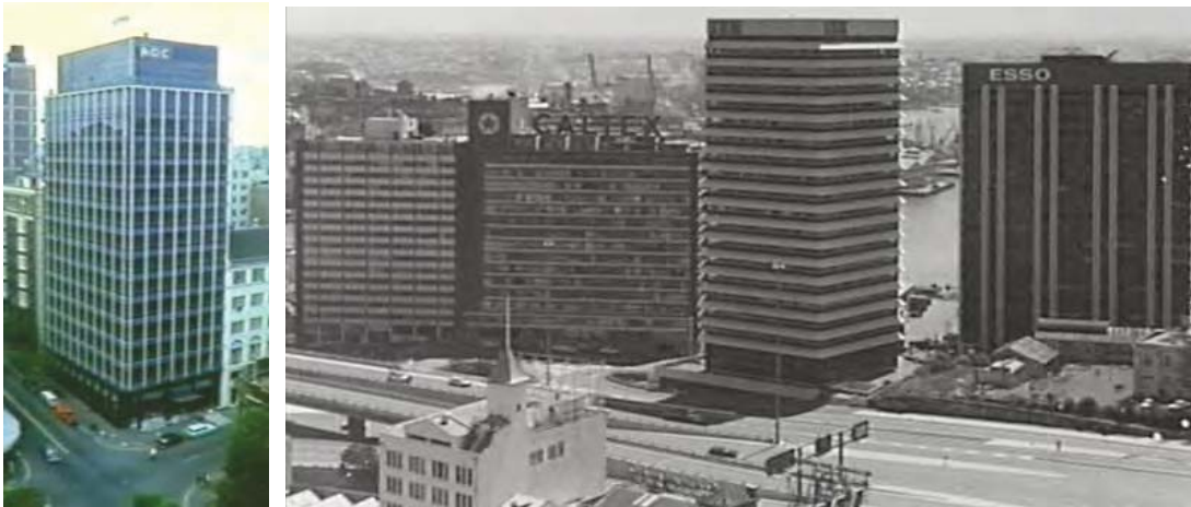
Figure 27 AGC House (left) and the IBM Building, dwarfing contemporaries: from left to right ADC House, 189-197 Kent Street, designed 1963-64; Caltex House; Esso Building, 137-153 Kent Street, designed circa 1967-68.
