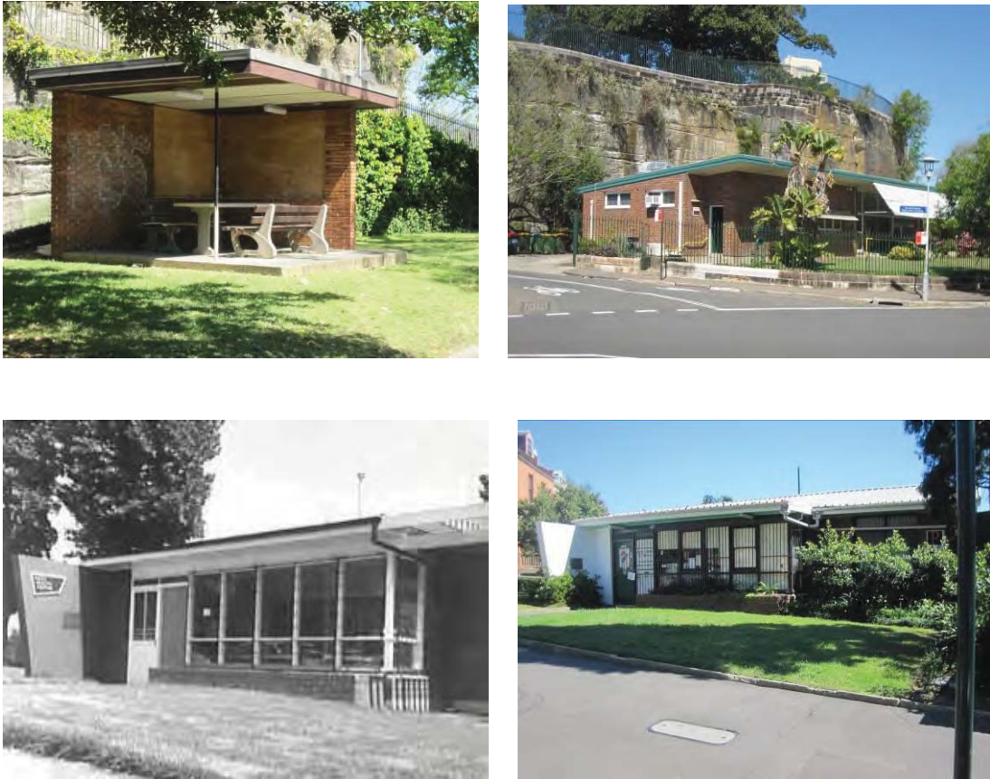
Figure 47 Group of community buildings and structures at Miller's Point constructed by the City of Sydney: a park shelter, the Harry Jensen Welfare Centre and the Lower Fort Street baby health centre, shown shortly after completion and in its present condition. Sources: TKDA; CSA SRC2574.
