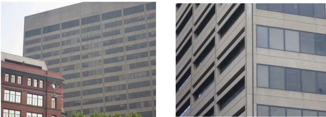
Figure 43 The clean flush finish of the McKell Building's principal southern facade (left), is in marked contrast to the northern facade, which was designed to control the impacts of the sun on the building's interior (right).
