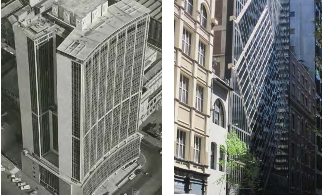
Figure 23 Two bold curtain walls: the gentle arc of the AMP Building (left) and the decorative geometries of 263-273 Clarence Street. Sources: SLNSW, PXA 907 Box 15, Ern McQuillan photograph (AMP); TKDA (263-273 Clarence Street).
