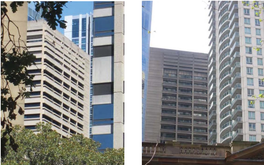
Figure 44 Precast concrete cladding and sun control systems on the northern and southern facades of the Water Board extension. Source: TKDA.
