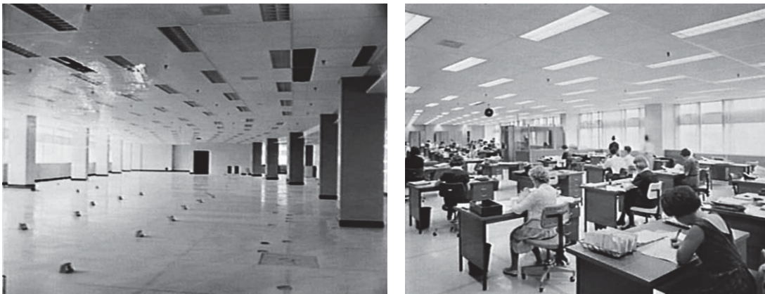
Figure 39 Office level of the AMP Building before and after occupation. The integrated and modular character of the ceiling system, lighting and services is apparent, as are the services installed at floor level. The photograph at right captures the quality of light, combining natural and artificial illumination. Source: SLNSW, Australian Photographic Agency – 11540 and 12113.
