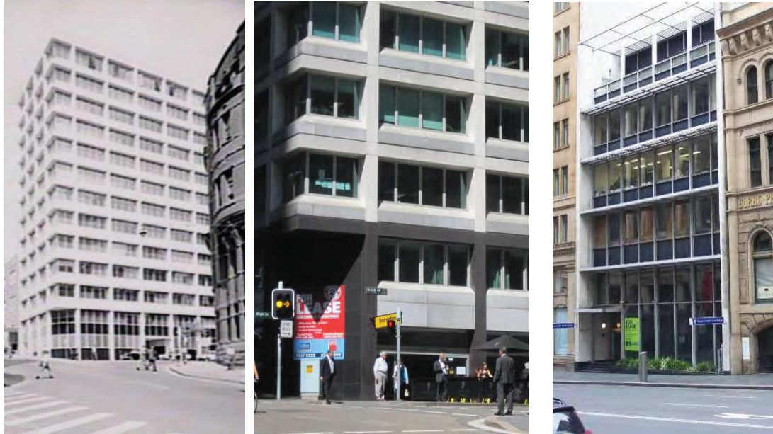
Figure 25 Temple House shortly after completion (left) and details of modifications to facades (centre); Liner House, which is substantially more intact (right).
