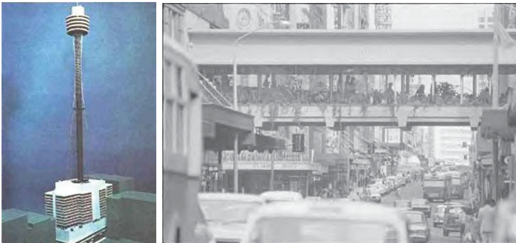
Figure 64 Centrepoint: model of the original scheme (left) and one of the pedestrian bridges associated with the development.
